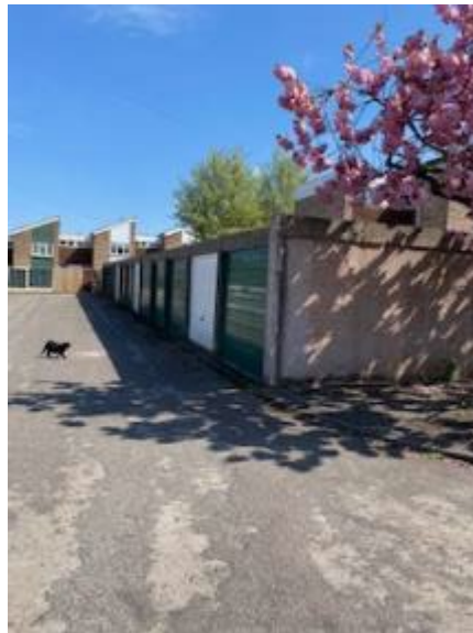
Garages to be demolished
