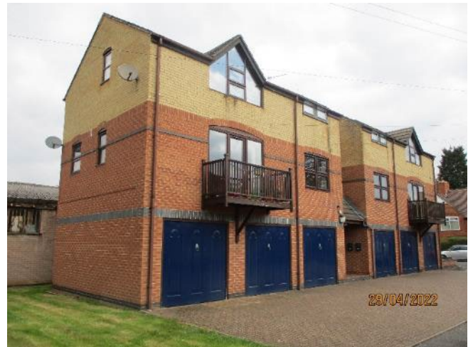
View from neighbouring block.
