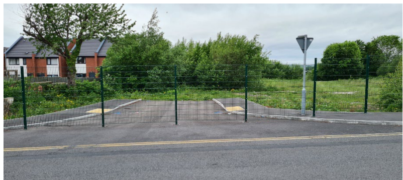
View of access/overgrown site
