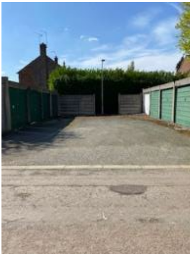
Garages to be demolished
