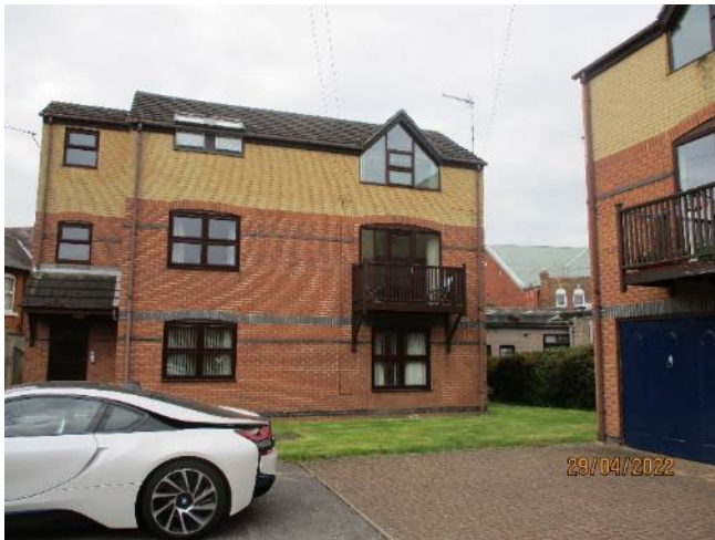
Neighbouring block to south west.
