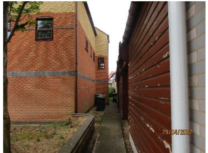
Rear north west elevation and boundary with industrial unit.
